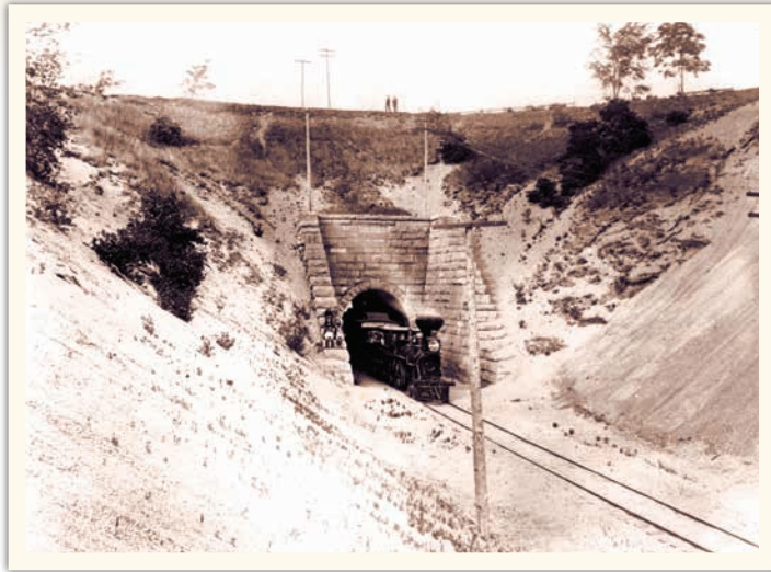
Two views of the railroad tunnel in Burlington, Vermont, built between 1860 and 1861. It is considered a testimony to Linsley's genius as an engineer as it had to be dug through loose sand 75- to 80-feet deep.
