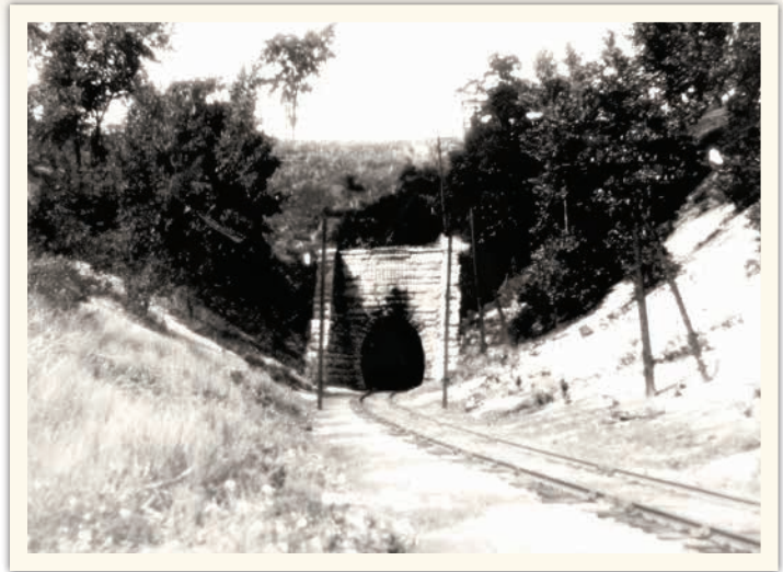
Two views of the railroad tunnel in Burlington, Vermont, built between 1860 and 1861. It is considered a testimony to Linsley's genius as an engineer as it had to be dug through loose sand 75- to 80-feet deep.
